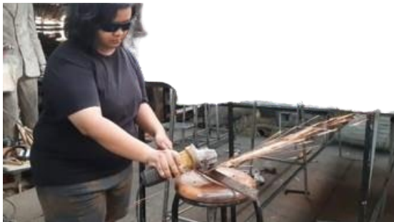
Figure 16. Material Preparation for Trusses (Source: Temanku Lima Benua, 2024)
