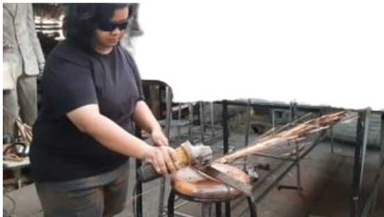
Figure 16. Material Preparation for Truses (Source: Temanku Lima Benua, 2024)
