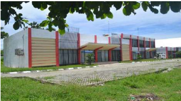
Figure 4. PIRNas building (Source: Zulyo's Documentation, 2017)
